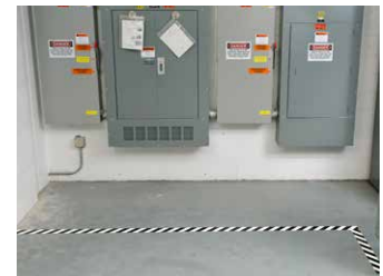
6. Colour-code areas in front of electrical panels.
