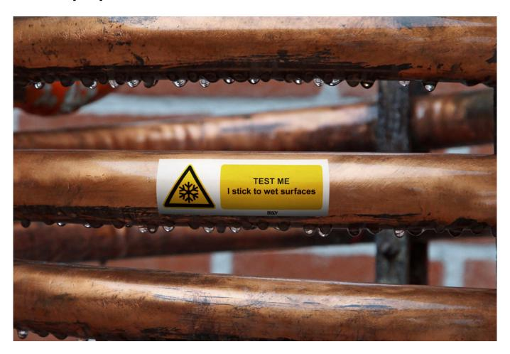
Wet and condensed surfaces are notoriously difficult to label in a reliable way. Labels tend to get saturated and fall off quickly. B-7530 however stays attached and remains legible. It is a polyester label that offers excellent adhesion to wet and condensed metal surfaces.
