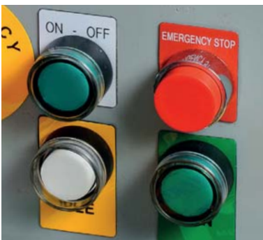
Control Panel Labels
