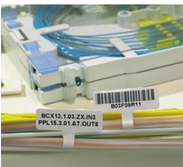
Fibre Optic Cable Markers
