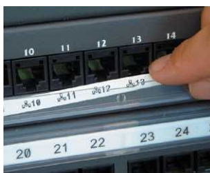
Punch block & patch panel labels
