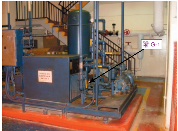
See Gate Valve identifier for exact location
