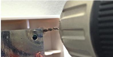
4. Position reader in mounting location and drill through guide holes.\*
