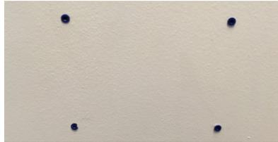
5. Use drywall anchors to secure in the wall.
