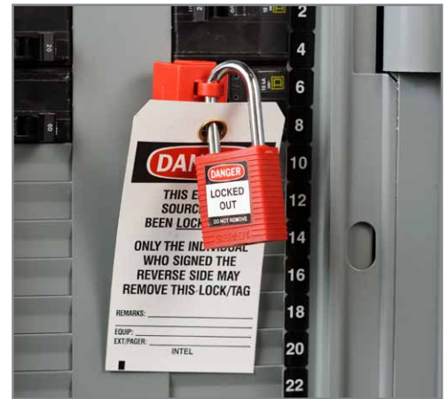
Using plastic-bodied padlocks, such as the Brady Safety Padlock, helps your employees differentiate between padlocks used for lockout/tags-plus purposes and general security purposes.
