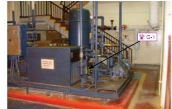
See Gate Valve identifier for exact location
