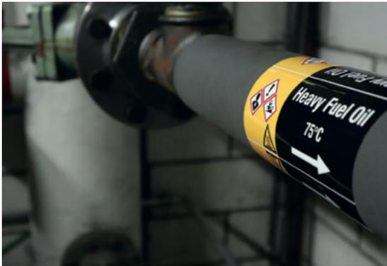
ISO 20560 pipe markers are globally recognized. The usage of pipe markers compliant to the ISO 20560 will increase your plant safety. Those pipe markers are a combination of 2 colour zones:
