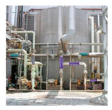
The usage of pipe markers compliant to the SANS 10140 will increase your plant safety. Those pipe markers are a combination of colours. In addition, pipe content legend and arrows can be shown. The colours to follow are indicated in the table below. The layout of the pipe itself with legend and arrows are up to the customer choice/standard.
