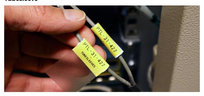
Well-identified cables offer an immediate insight into how an installation works and how it is connected. The non-adhesive Tubesleeve enables cable identification that stays in place and can be rotated at the same time for fast updates and repairs with a reduced risk of human error.
