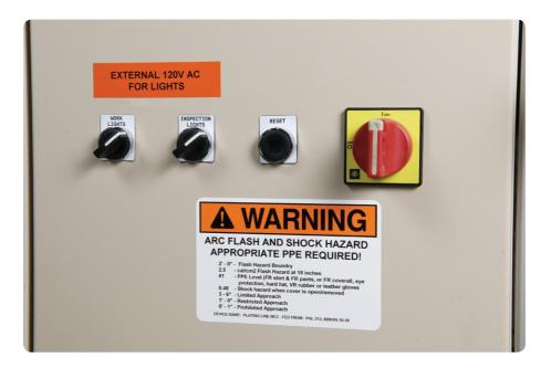
Arc flash has the potential to cause substantial damage, fire or injury. Clearly visible and legible warning labels should be positioned in the arc flash hazard zone to prevent injuries. Other prevention measures include appropriate usage of arc flash personal protective equipment (PPE), remote equipment operation or reconfiguration of electrical equipment.
