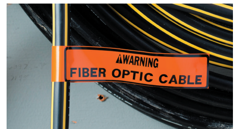
Fiber Optic Cable Markers
