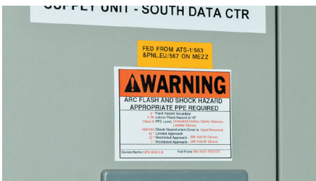
Arc Flash Services and Labeling
