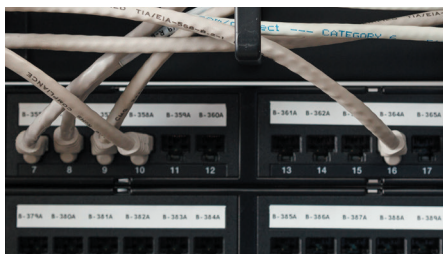
Patch Panel Labels
